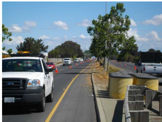
Maintenance of Richmond Parkway Medians
