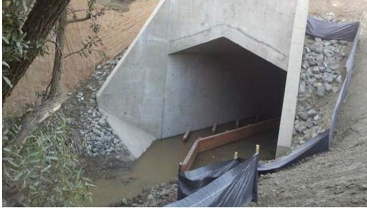
**Upstream Headwall:** The “Headwall,” or upstream receiving end of the culvert, is visible in this photo. Wooden baffles were installed in accordance with environmental regulatory requirements. The baffles encourage sediment deposit and development of water eddies, mimicking a natural stream, enabling flora and fauna to thrive, and ultimately promoting a healthy riparian ecosystem.
