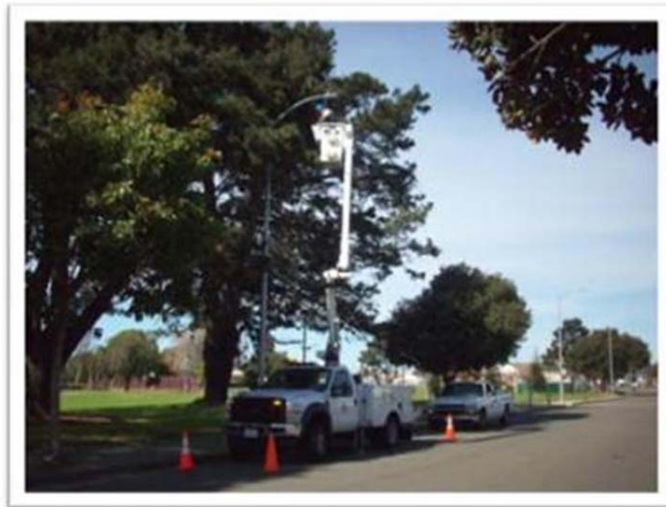
Electricians repairing a street light at John F. Kennedy Park
