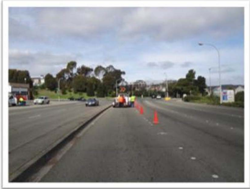
Button Installation on Hilltop Drive
