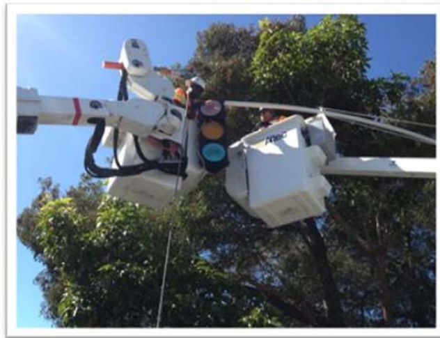
Installation of Wiring on Carlson Boulevard
