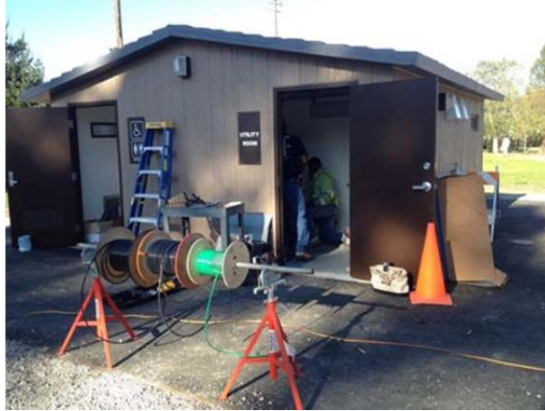
Power Installation at Booker T. Anderson Restroom Facility
