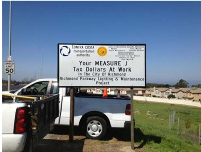
Installation of Measure J Sign
