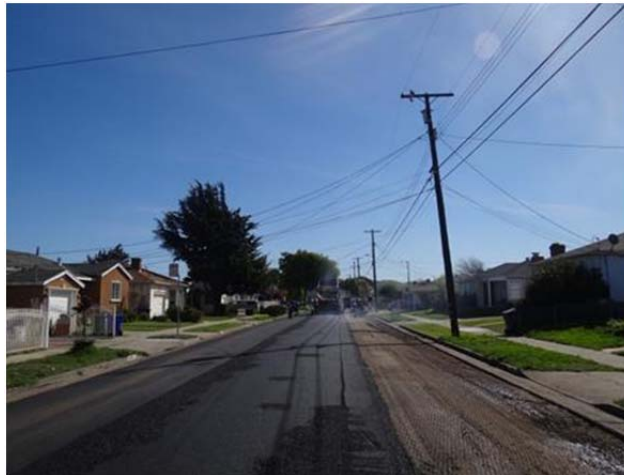
Paving on Hellings Avenue
