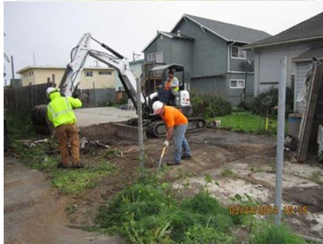
These pictures show the same lot before and after demolition work.
