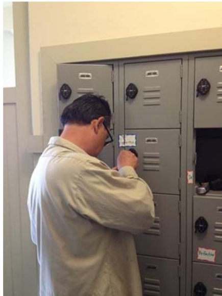
Repairing Locks at the Plunge
