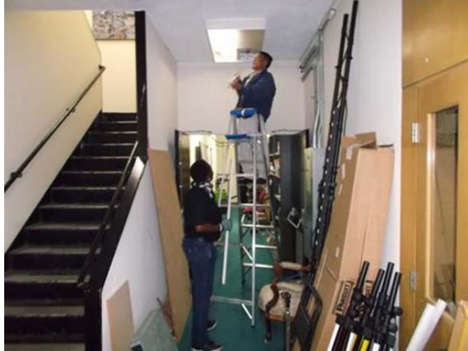
Replacing Lighting Tubes and Covers
