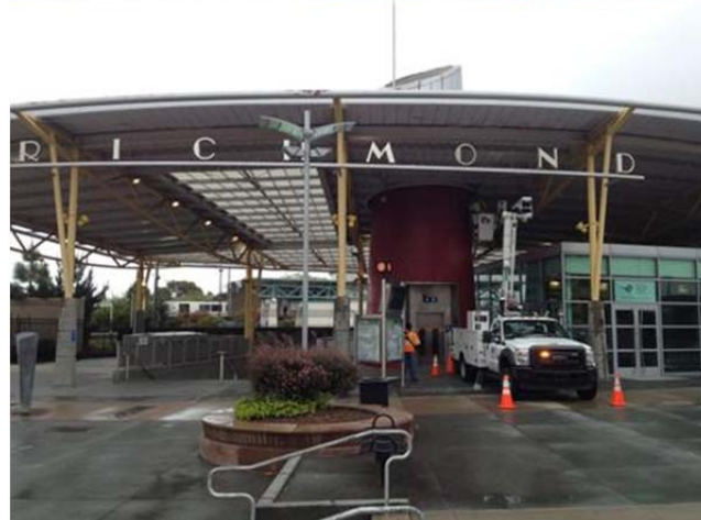
Repairing Lighting at the Richmond Transit Center
