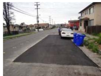
Dig Out – Ripley Avenue
