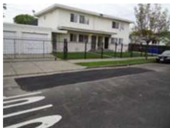
Dig Out – 2 nd & Chanslor Avenue
