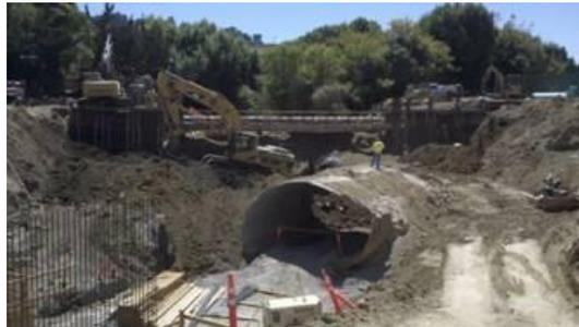
The last remaining portion of the corrugated metal pipe culvert is visible in the center of the above photograph; in the background is the 36" sewer line suspended in the truss that was originally suspended over San Pablo Creek, and in the lower left corner the rebar for the new concrete culvert is visible.
