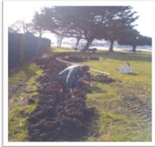
Trenching Off of Richmond Parkway
