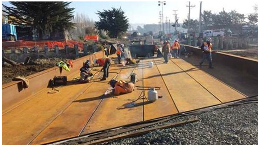
9:30 am Sunday, December 15 th , bridge in place, deck plates being welded
