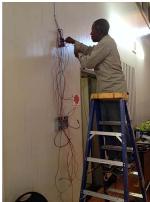
Light Switch Relocation at Booker T. Anderson
