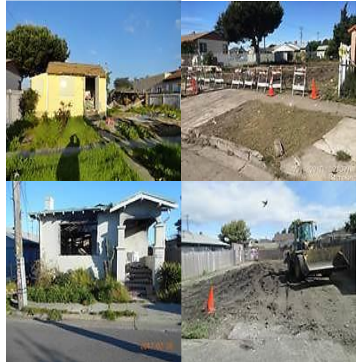
Before and after – abandoned properties are demolished
