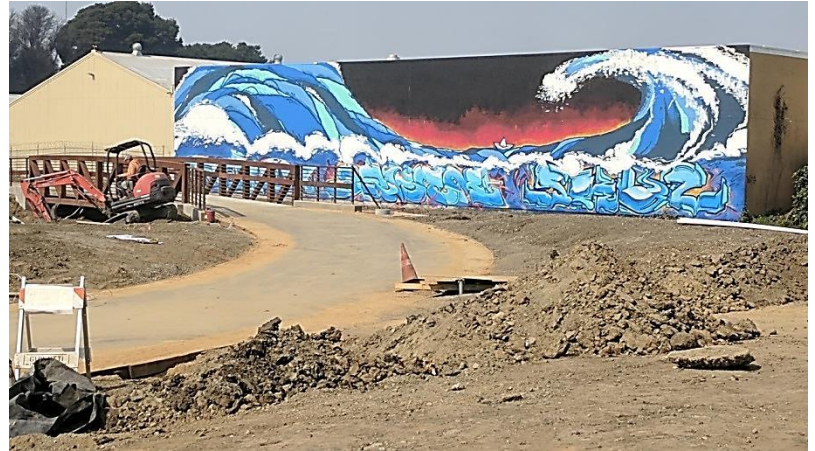
The Greenway Gap Closure Project at San Pablo Ave
