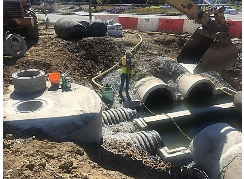
Hydrodynamic Separator Installation
